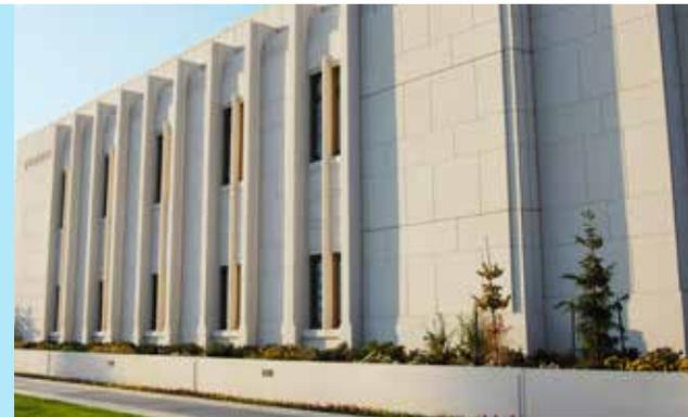
Dimensions of the structure are 178 feet, 10 inches by 87 feet, 10 inches. The exterior walls of the 31,245-square-foot building are made of precast concrete panels with a quartz rock finish that weigh up to 30 tons. The quartz rock was mined in Washington state.
