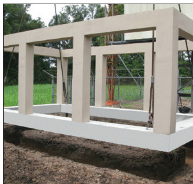
Placing The Chain Wall
