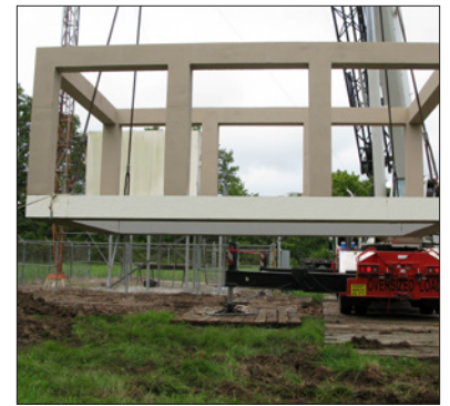
Lifting The Chain Wall
