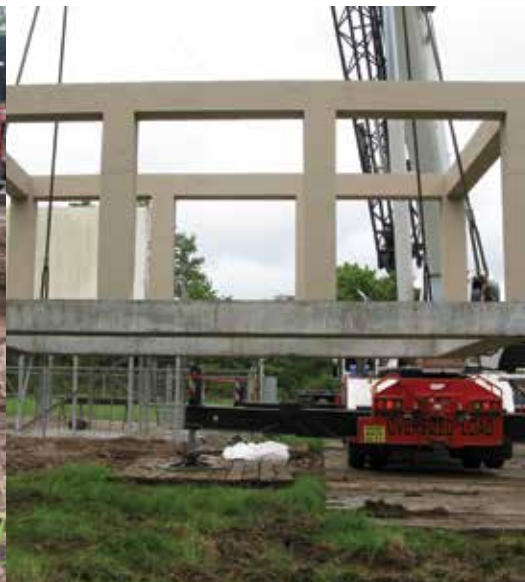
Lifting the Chain Wall
