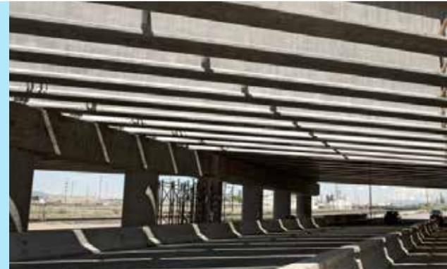
At 198 feet, 10 inches in length, the bridge also features the longest prestressed concrete bulb 'T' girders used up to that time by UDOT. The girders were produced by Forterra at their Salt Lake City facility.
