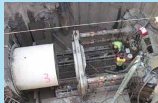
Jacking station: PM-13 shaft
