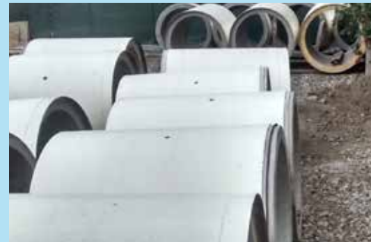
PM-13 Site: delivered 72" RCP for Curved Microtunnel
