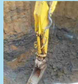
PM-13 Shaft Excavation
